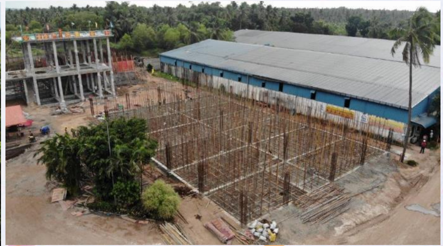
Engineering & Power Centre
