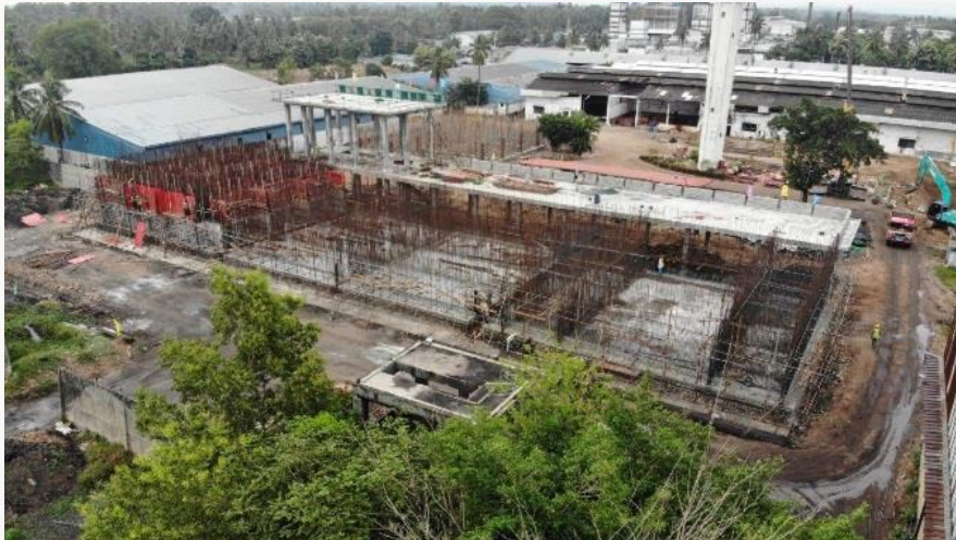
Effluent Treatment Plant
