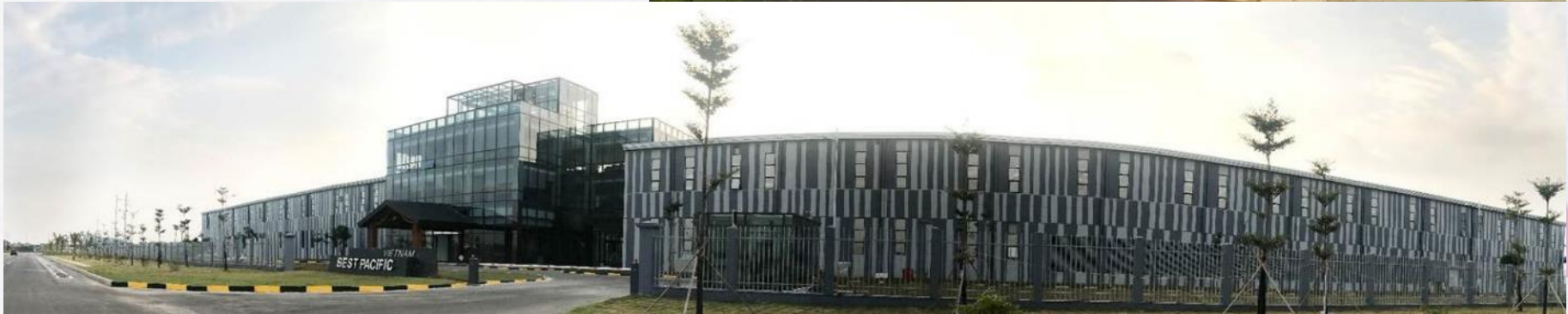
Overall site (side view)
