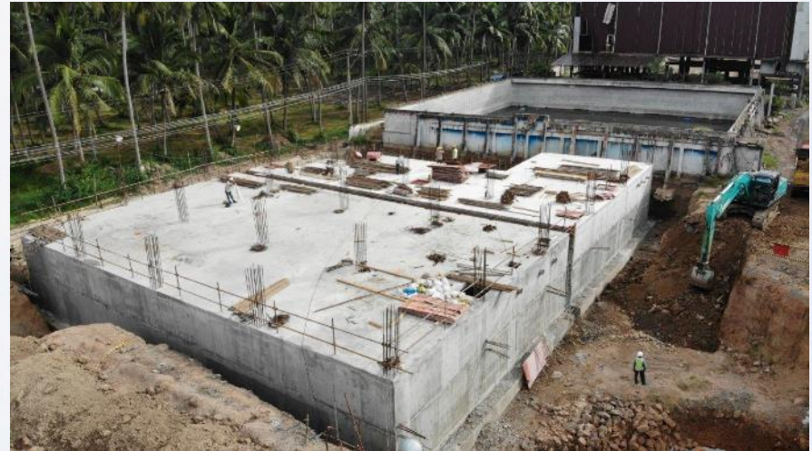
Rural Water Treatment Plant
