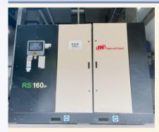
Replacement of the old single-stage air compressors with new permanent magnet two-stage compression air compressors
